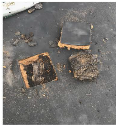
Roof cut performed to determine it's composition
